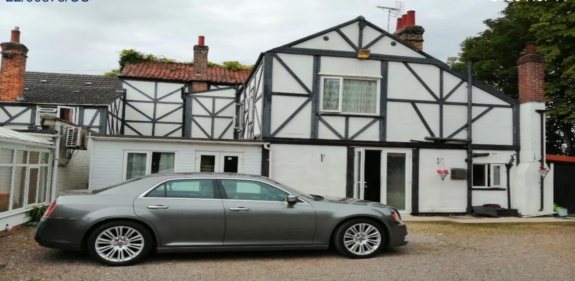
Rear/north view of the property
